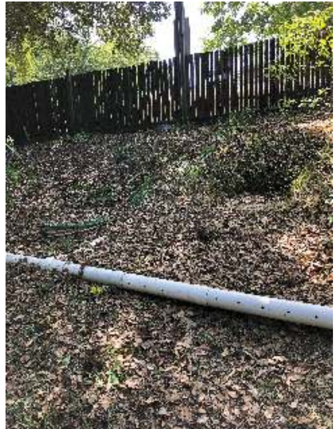
Perforations in the grey-water pipe allow us to send our laundry water back into the ground for plants.
