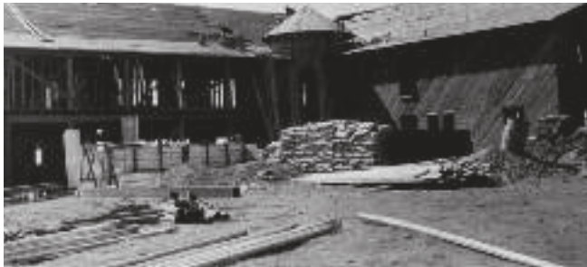
The Ranch House under construction circa 1930.
